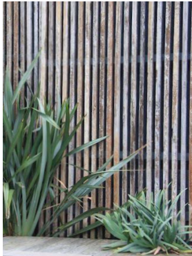
Hardwood Batten Screens
