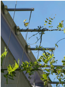
Vertical SS Wiring
